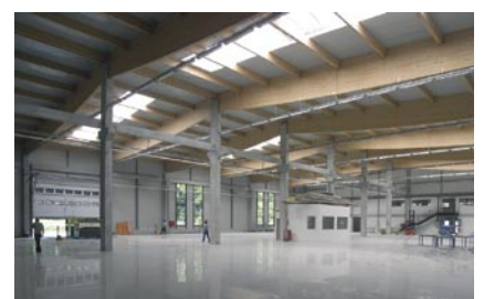
Interior view: Hronská Breznica
